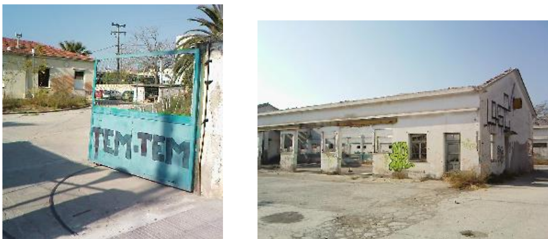
Figure 3: The main gate (left) and an underutilized building (right) (Source: photos taken by the author)
