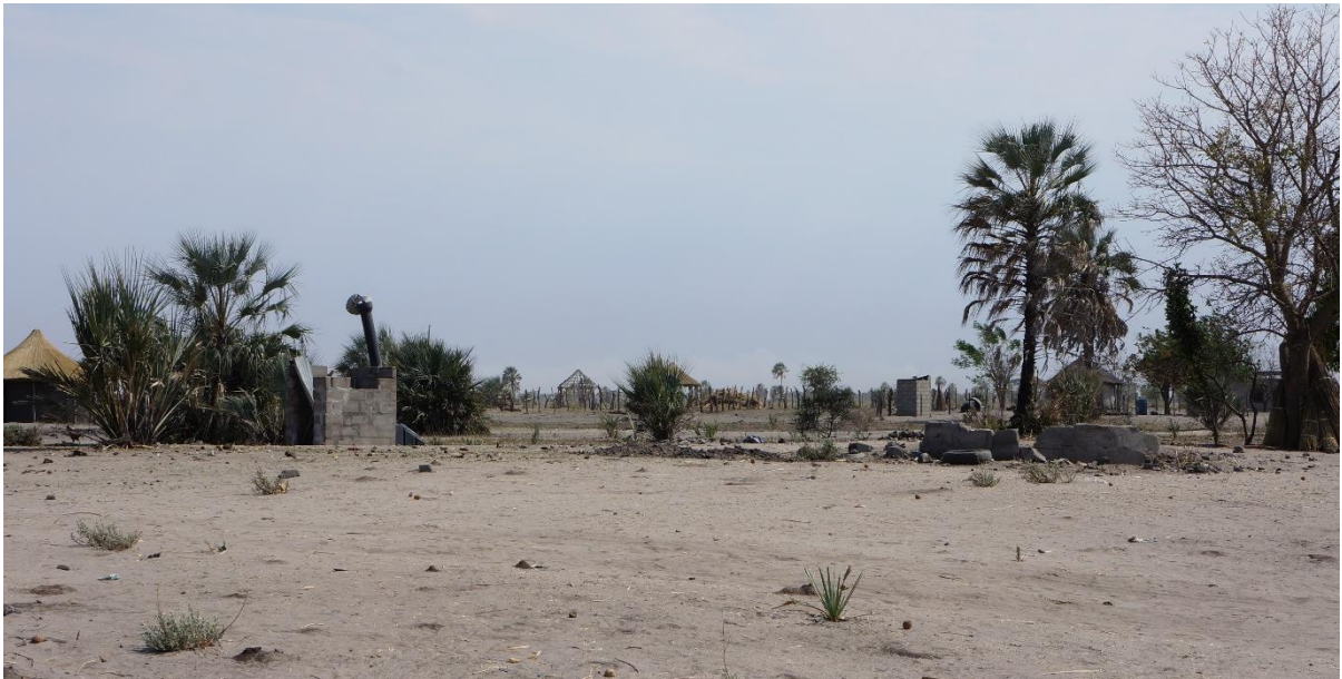
Figure 5. Houses that were destroyed by the previous floods in Tubu.
