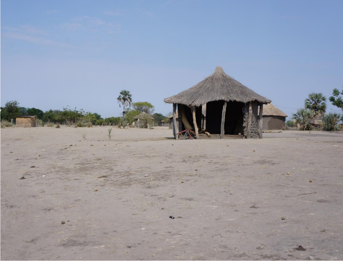
Figure 13. A house destroyed by the flood.
