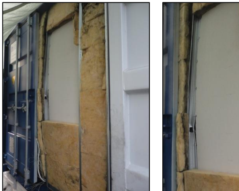
Figure 13. Collapsed inner wall at cargo opening
