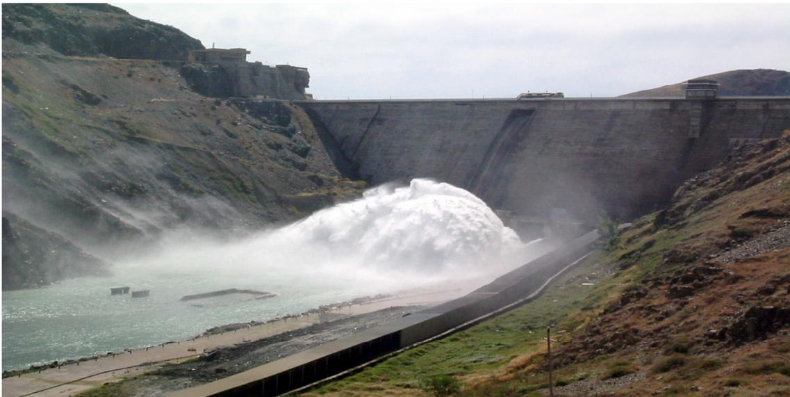
Figure 2: Pictorial view of 84 m high wall and discharge point of Talas Dam. The dam was constructed in 1975 (Rasskazchikov 2010). Image source (CTWC 2008)
