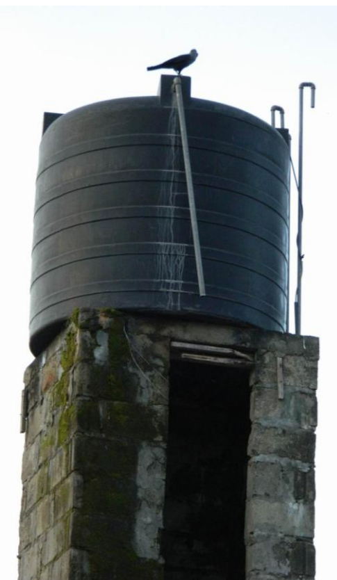
Fig 4.15 The most common type of water tank
