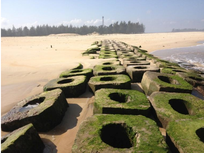
Figure 6:5 The groin at Thuan An inlet, photo taken from the end of the groin towards the shoreline. Picture of the beach and the groin at the same height, showing the groin to be permeable (Photo: Eva-Lena Eriksson).
