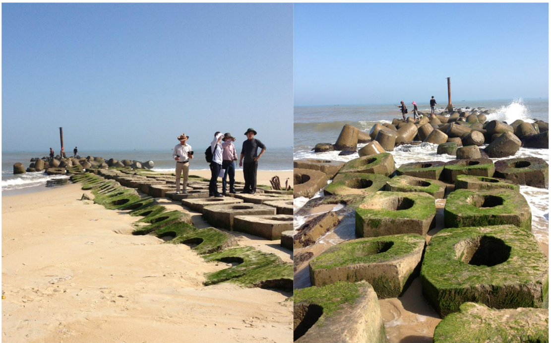
Figure 4:17 Groin at Thuan An inlet, January 2013 (Photo: Eva-Lena Eriksson)
