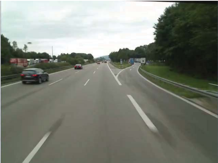
Figure 8 Screenshot from Front View Camera Recording Showing Highway Exit. The problematic part of this situation is the guard rail on the right side of the road trailing off with the exit. The new position of the guard rail, closer to the road, must be identified when the vehicle has passed the exit.
