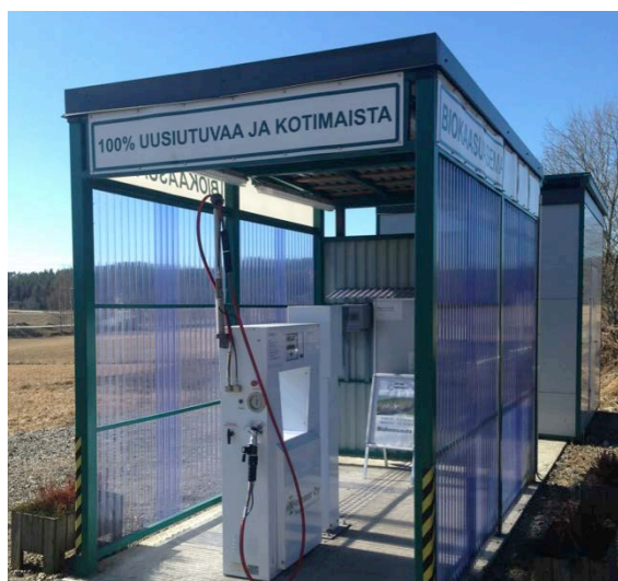
Figure 9 Biogas vehicle fuelling station
