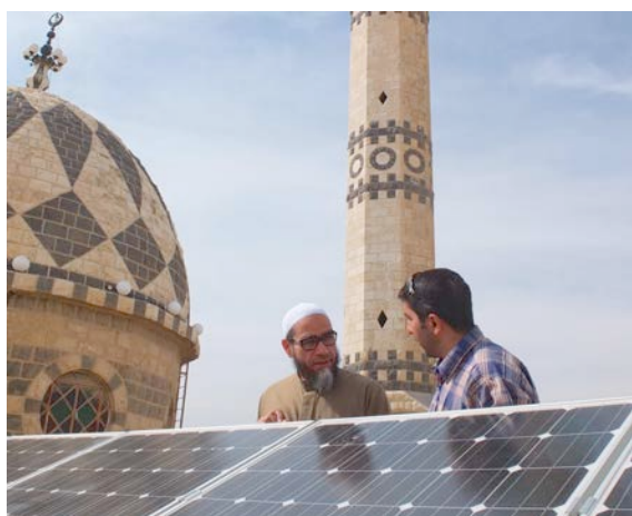
Figure 3, Solar PV installation at Mosque Abu Darwish, Amman, Jordan. Photo: Håkan Rodhe, IIIIEE.
