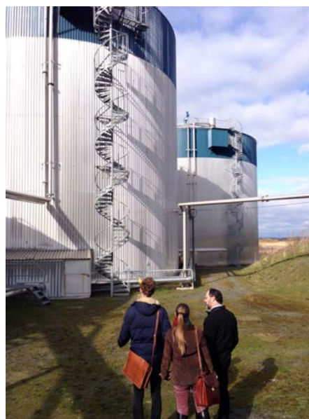
Figure 2: Karpalund Biogas Plant
