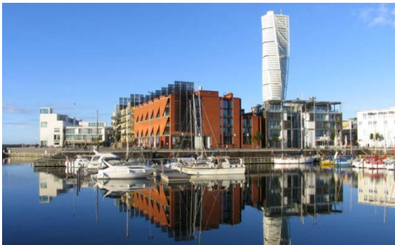
Figure 7. Bo01 development in Malmö, Sweden (Source: Malmö stad).
