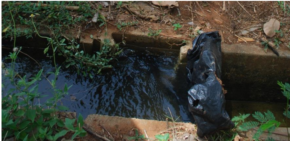
Figure 5:1. The irrigation water supplied to farmers cultivating different crops is regulated by canals such as the one seen in the figure. In this picture a pipeline is connected to the canal, which leads the irrigation water to the field. In this figure the pipeline is connected to the canal just before the water is blocked. The water is regulated, according to a schedule, by the farmers themselves. Photo: Erica Perming, 2009.
