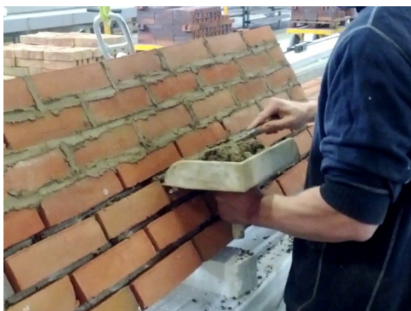
FIGUR 7.4: Fogning mellan skärvor
