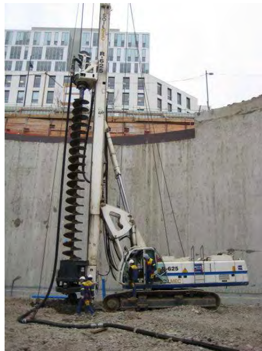
Picture 11 : Piles achievement
