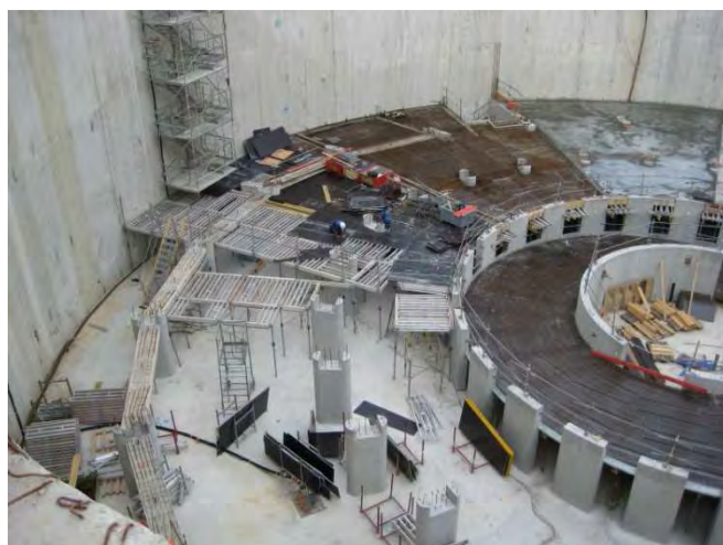
Picture 14 : Achievement of the floors slabs
