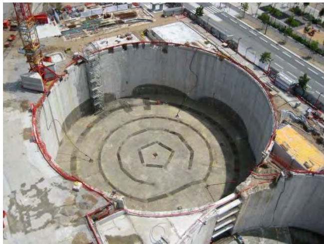
Picture 13 : Achievement of the bottom slab
