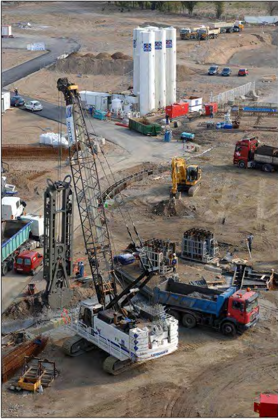
Picture 8 : diaphragm walls digging
