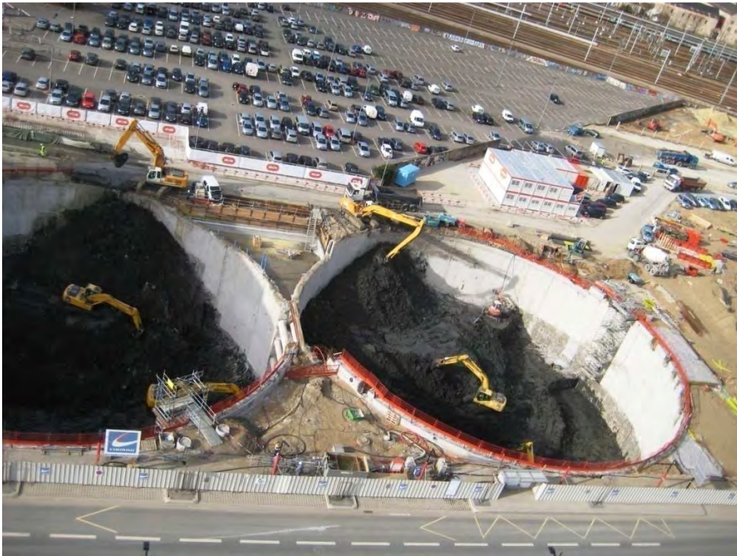
Picture 10 : Soil digging inside diaphragm walls
