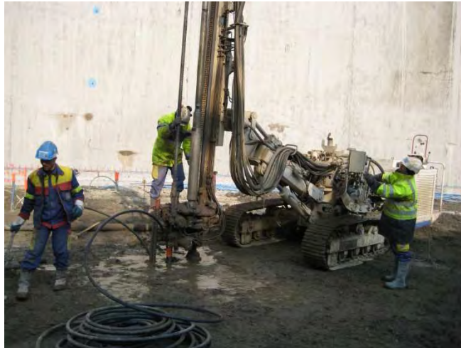
Picture 12 : Achievement of micropiles
