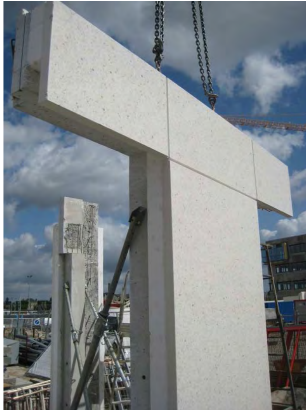
Picture 25 : example of sandwich element
