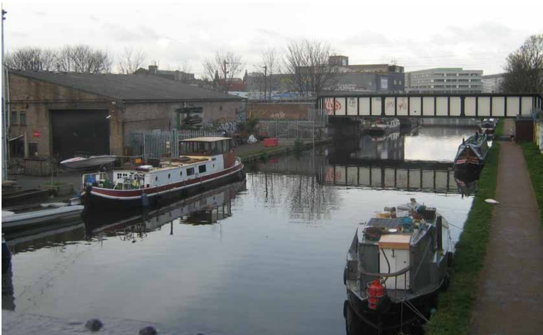
Figure 9. Photograph of Lea Navigation Canal regeneration near Hackney Wick. Source: Personal Picture
