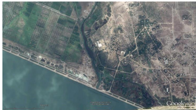
Figure 4 Maga dam, Source: Google Earth accessed 2014-05-19
