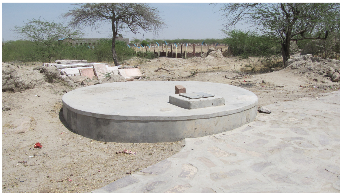
Figure 6. A tanka that can only be refilled because it has no inlets. Photo: by author.
