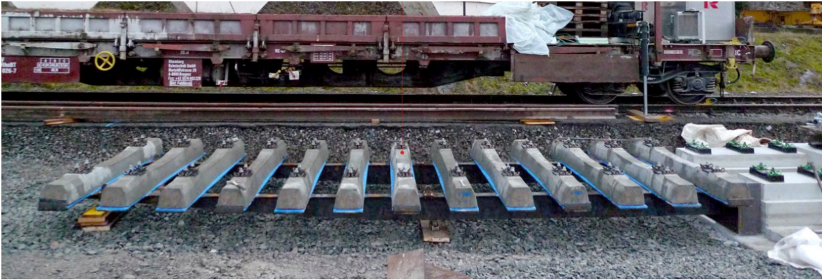
Figure 19. The universal transition module V-TRAS pictured as it is provided and supported on the massive end of the ballastless track and floating in the ballast bed (Rohmberg Rail, 2013).
