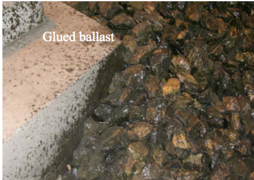
Figure 10. Glued ballast (Xin, Kumar & Gao, n.d.)
