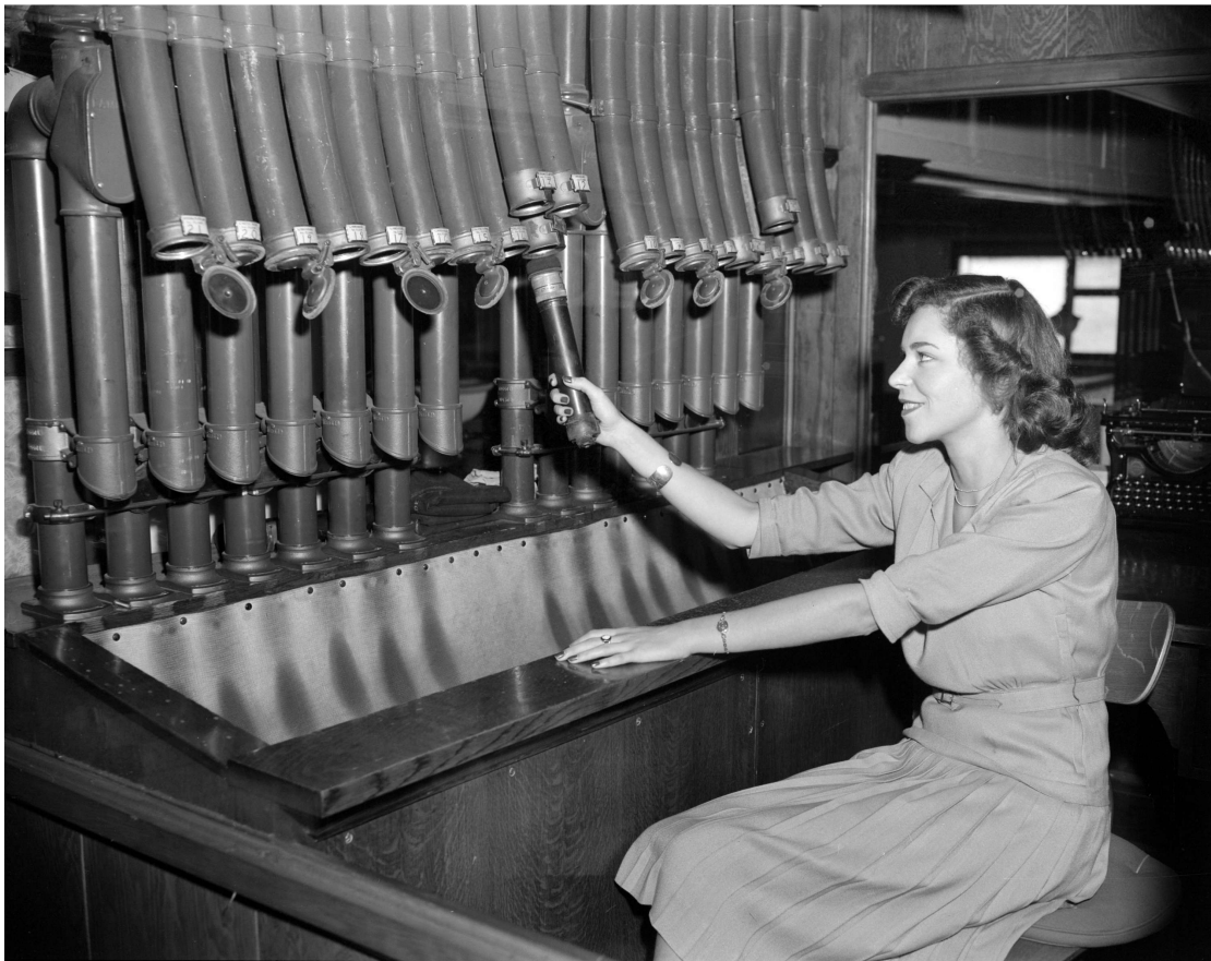
Figure 4. Woman using pneumatic tube delivery system in Vancouver, Canada (Image: Photo by Jack Lindsay, 1946).
