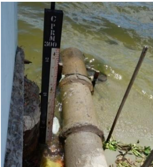
Figure 17. Untreated sewage discharged directly into the lagoon.
