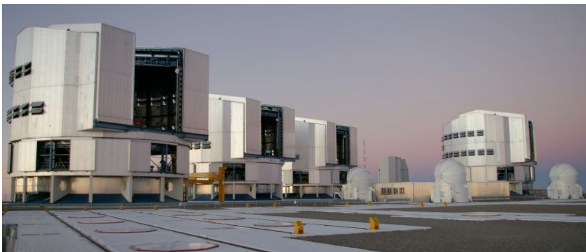
Figure 1.5: VLT on Paranal, the 4 large UT's can be seen and 3 of the 4 AT's, image from ESO.
