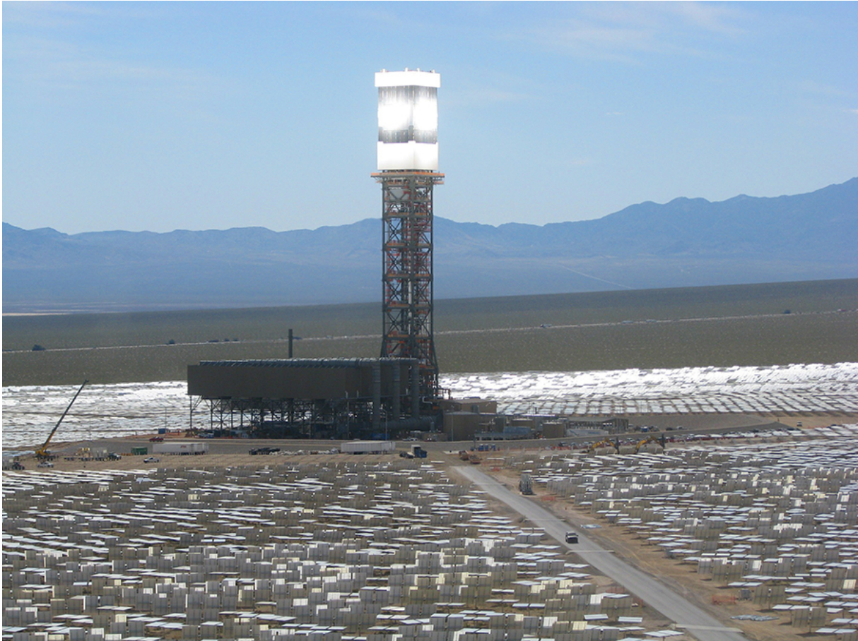
Figure 3 BrightSource Ivanpah central receiver and heliostat field under construction. [8]
