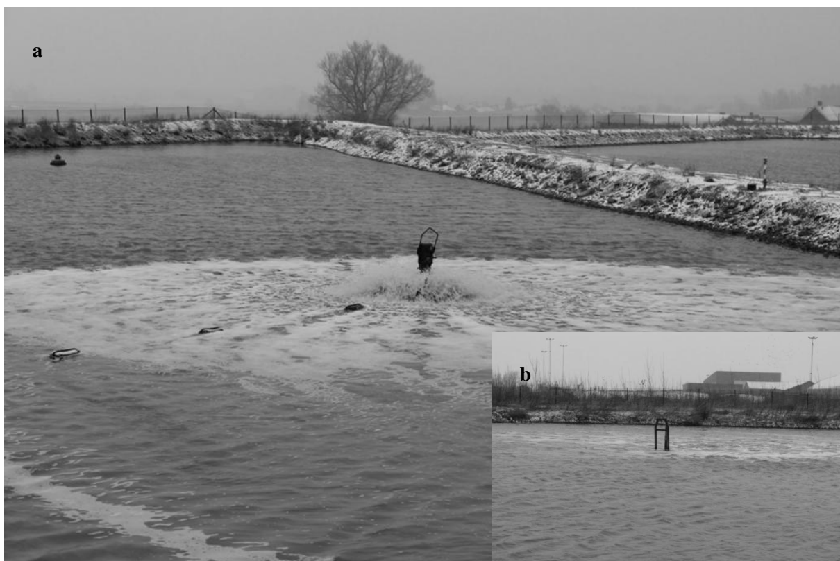
Figure 4.1. Example of aerated lagoons in Hedeskoga landfill: a bottom aerator (b) and a surface aerator (a). Pictures taken with permission of Sysav. Author: Alessandro Sarno, Lund University.
