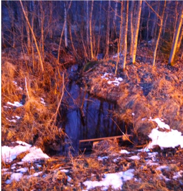
Figure 18: Current connection of the storm water ditch from rural areas to the urban sewer system.
