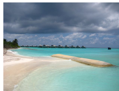
Figure 13. Geotubes installed by Seamarc
