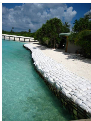
Figure 14. Sea wall of sand cement bags
