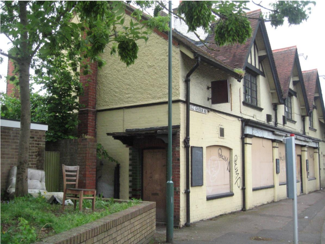
Figure 6: Photograph of derelict building perpendicular to London Road. (Taken by author, 2013)
