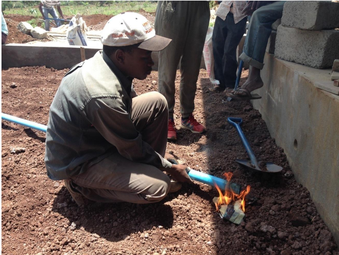
Fig. 4.32. Fire was used to make the material soft before connecting the pipe lines for the plumbing.
