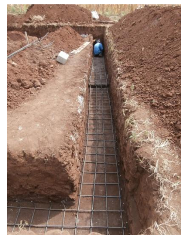
4. Fig. 4.11. Foundation footings with reinforcement.
