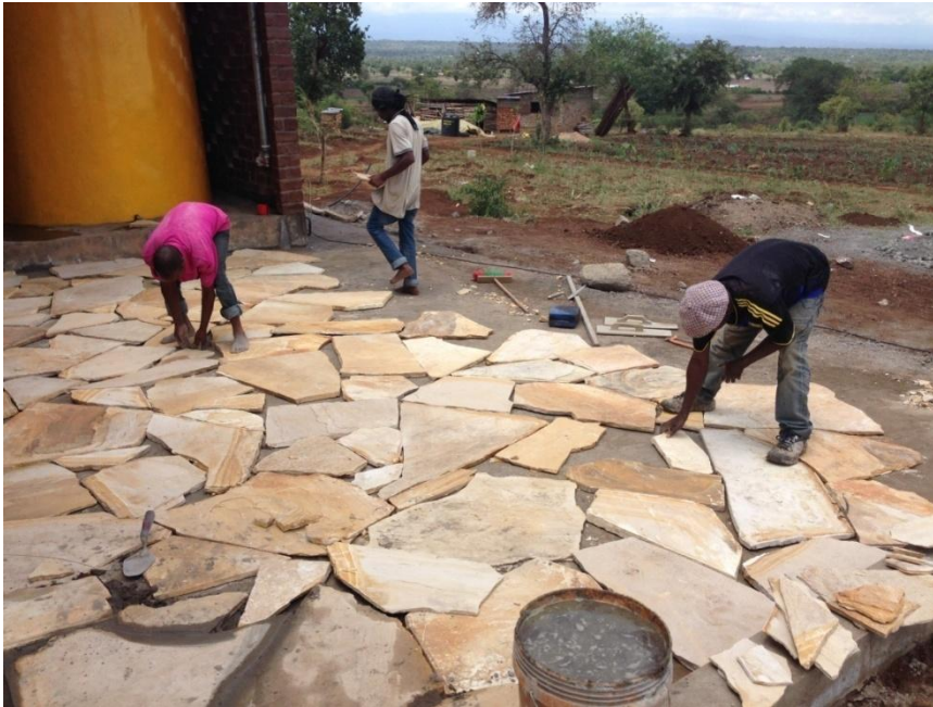
Fig. 4.35. Paving stones around the house.
