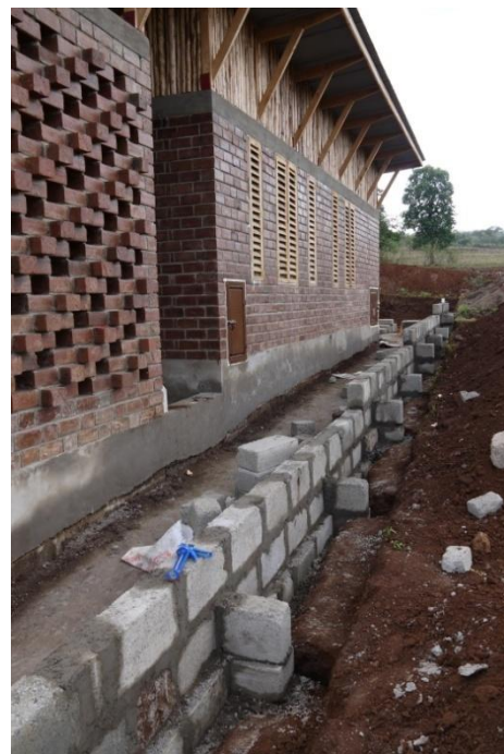
Fig. 4.34. The process of the brick wall around the house.
