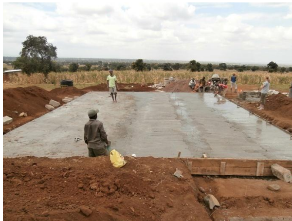
7. Fig. 4.14. The concrete foundation is ready.
