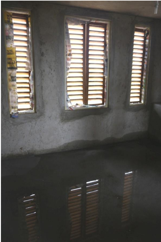
Fig. 4.29. The floor got watered to avoid cracks in the concrete.
