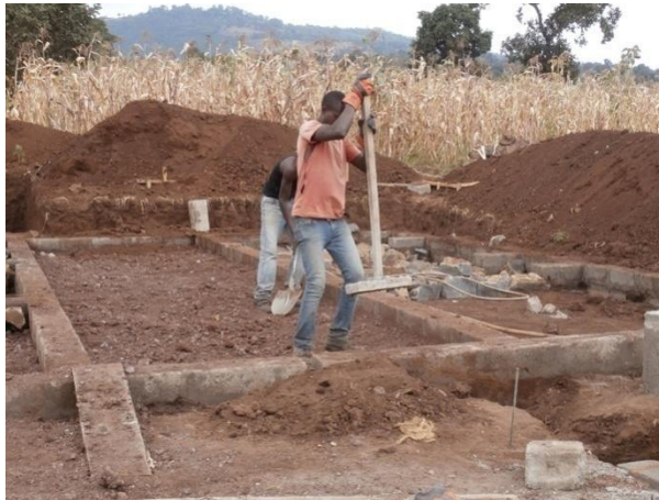
5. Fig. 4.12. Compacting the ground.
