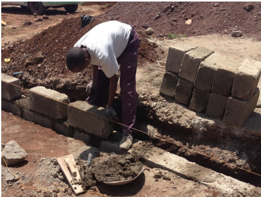
Fig. 4.31. The brick wall around the house is taking place.
