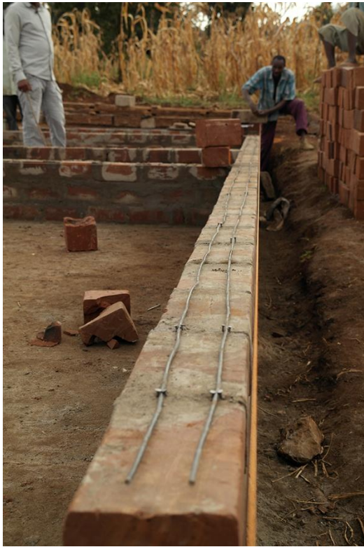
5. Fig. 4.19. First layer of reinforcement in the walls.
