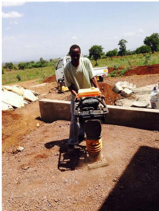
Fig. 4.33. A ground vibrator was one of few machines that was rented. Almost everything else was made by hand by using simple tools.
