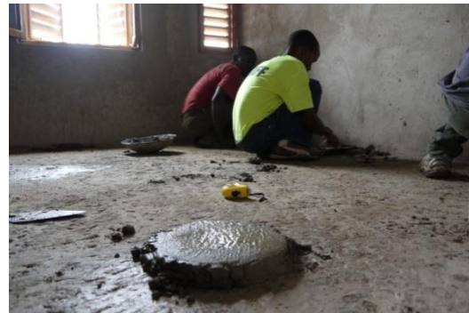
Fig. 4.26. Reference highs of concrete were placed to help the casting.
