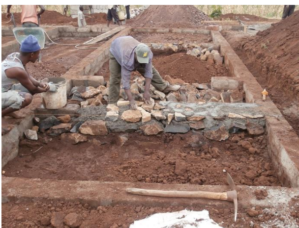
3. Fig. 4.10. Foundation of stones was settled under the inner walls to save material and cost.
