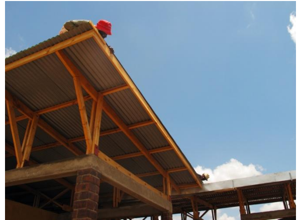
2. Fig. 4.23. The roofing sheet was attached to the trusses.
