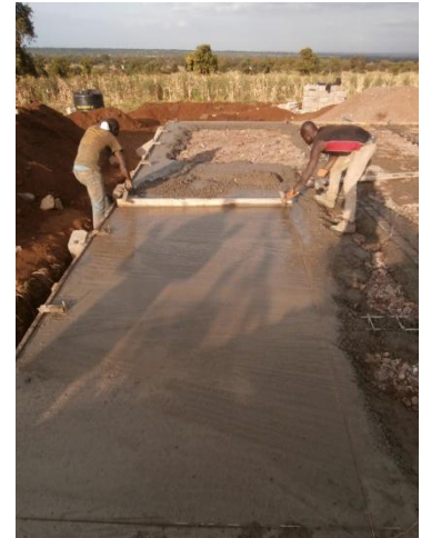
6. Fig. 4.13. A wooden board was used to level the concrete.
