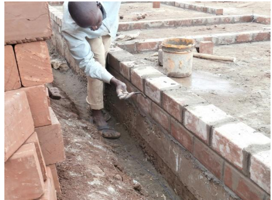
2. Fig. 4.16. A measure stick was used to get the right distance between the bricks.
