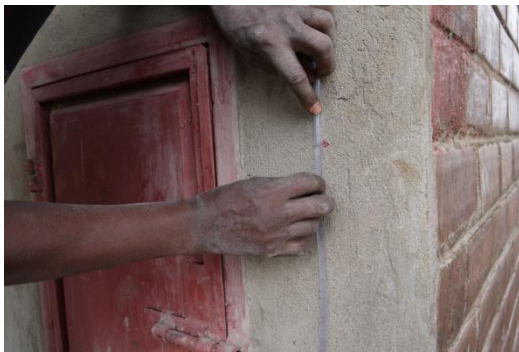
Fig. 4.25. Simple methods were used to find reference points before casting the floor.
