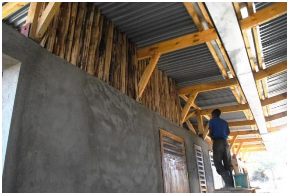
3. Fig. 4.24. Sisal poles were placed to fill the gap between the walls and the roof. They look natural to the house and also give good ventilation. The picture also shows the construction of the rain gutter that leads across the roof.
