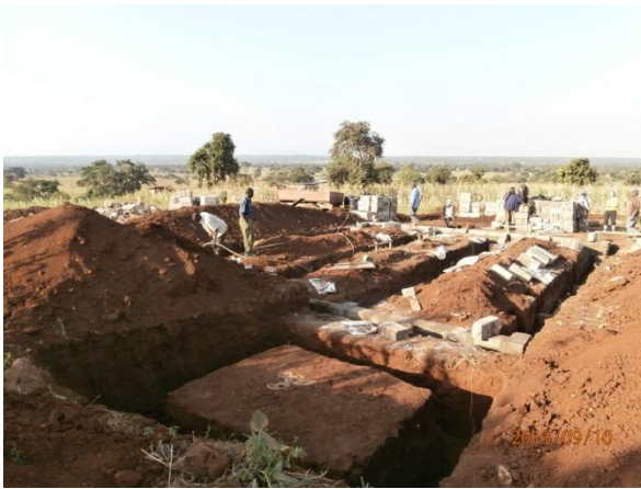
1. Fig. 4.8. Excavating for foundation.
