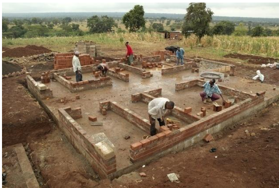
3. Fig. 4.17. The walls were put in place.
