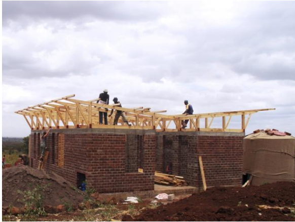
1. Fig. 4.22. The trusses were put in place. The inward slope design support the rain water collection and leads the water to the two water tanks placed on each side of the house.
