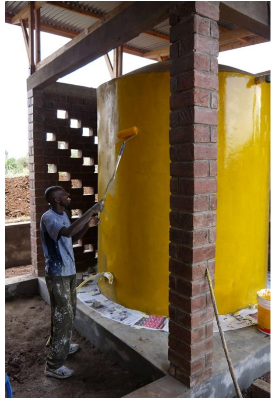
Fig. 4.30. One of the water tanks got painted.
