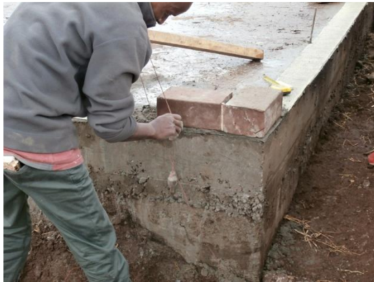
1. Fig. 4.15. A brick string and a level was used to get the first brick layer right.
