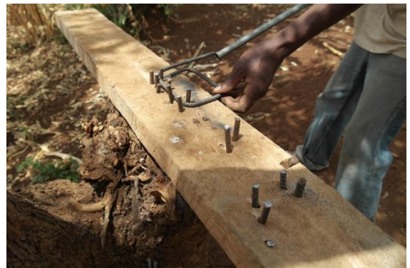
4. Fig. 4.18. Simple methods were used to bend the reinforcement bars.
