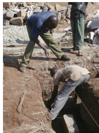
2. Fig. 4.9. Measuring of the foundation.
