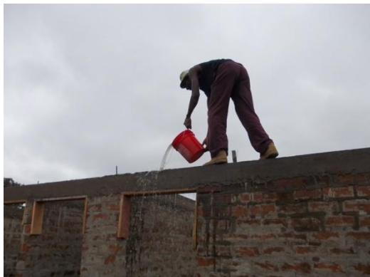
7. Fig. 4.21. The concrete of the ring beam got watered to avoid cracks in the concrete.
