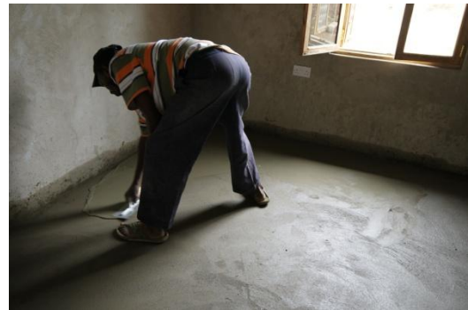
Fig. 4.28. The last finish of the floor casting.
