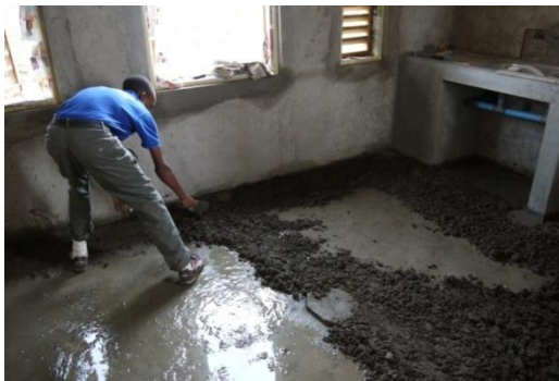
Fig. 4.27. Casting the floor.
