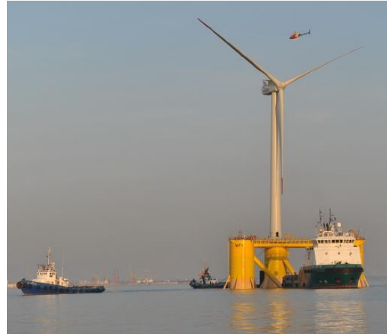
Figure 37. Towing to installation site of the pre-assembled WindFloat turbine. [85]
