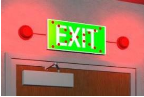
Figure 10. Sign 8: green background, EXIT text, LED X-marking, red flashing lights.
