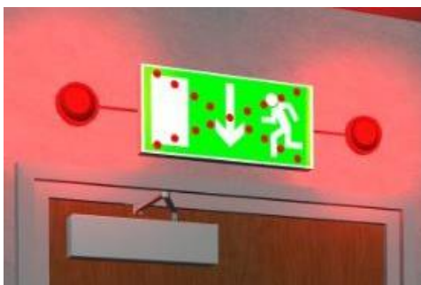
Figure 9. Sign 7: green background, running man pictogram, LED X-marking, red flashing lights.
