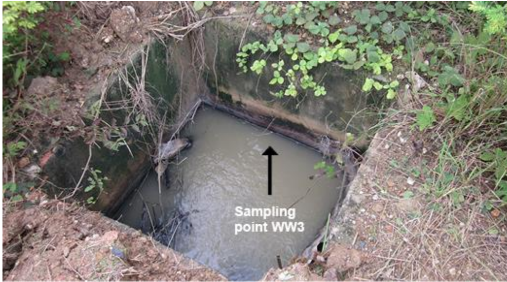
Figure 4.3. Sampling point for WW3. The photo is of WW3b, taken during the second visit to the factory. The concrete boxes look the same for WW3a and WW3c, with more or less soil filling the box. It should be noted that the colour of the water was darker than this during the third visit.
