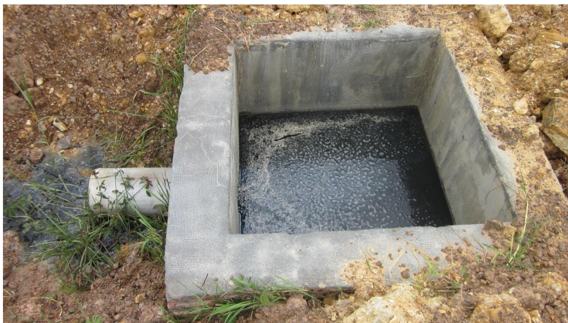
Figure 5.6. Concrete box for accessing the outlet from the anaerobic ponds. This photo was taken on the outlet from Anaerobic digestion 2 before construction was finished. The pipe to the left in the figure was later connected to the pipe directing the water to Pond 1, and covered with soil. The inlet to the box, meaning the outlet from Anaerobic digestion 2, is to the right in the figure but can not be seen as it is underground.
