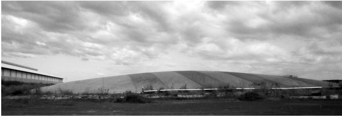
Figure 5.7. Photo of Anaerobic digestion 1 during the third visit to the factory. The grey HDPE canopy covers the whole pond to create a gas storage.
