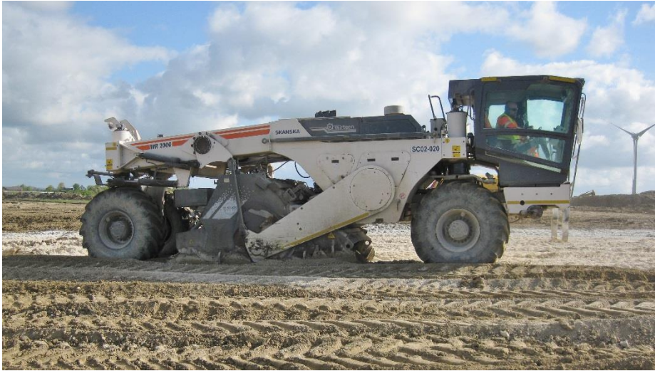
Figure 2.6 A machine mixing the lime with the soil at ESS.
