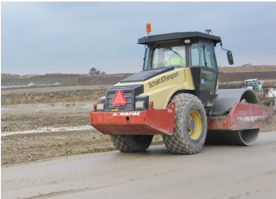
Figure 2.7 Compaction work with a vibrating smooth drum at ESS.
