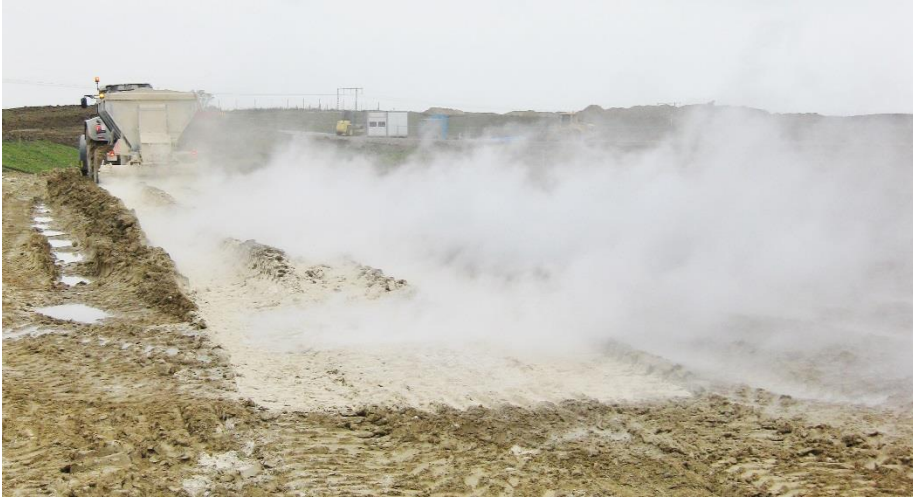
Figure 2.8 Steam rises due to the exothermic reaction which occurs between quicklime and the water in the soil.
