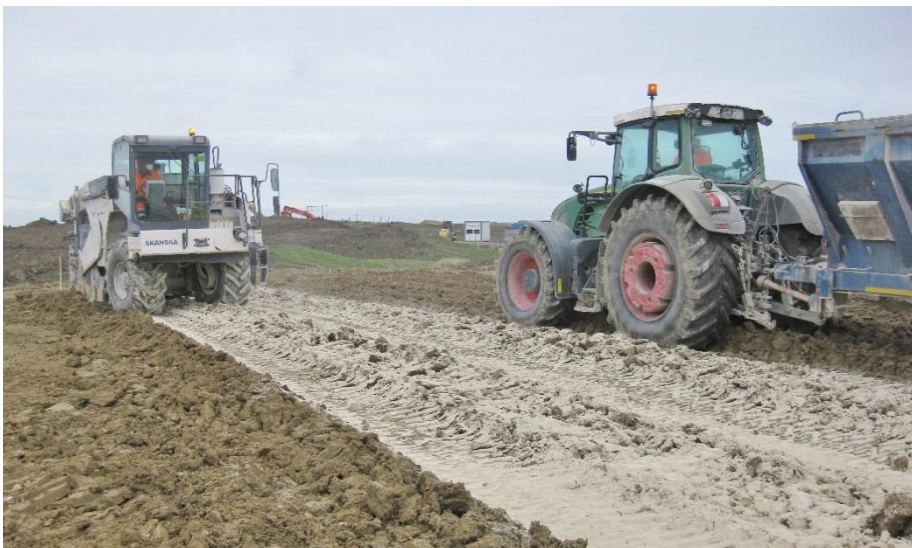
Figure 4.3 Ongoing modification at ESS.
