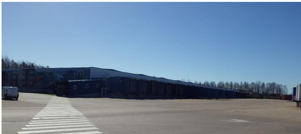
Figure 8. House 3, DC North (Photo Eliasson).
