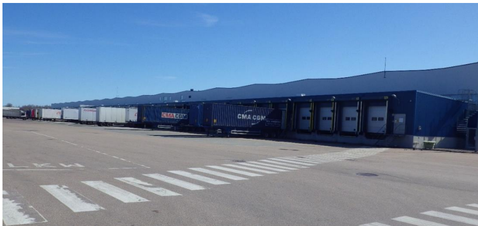
Figure 7. House 2, DC North (Photo Eliasson).
