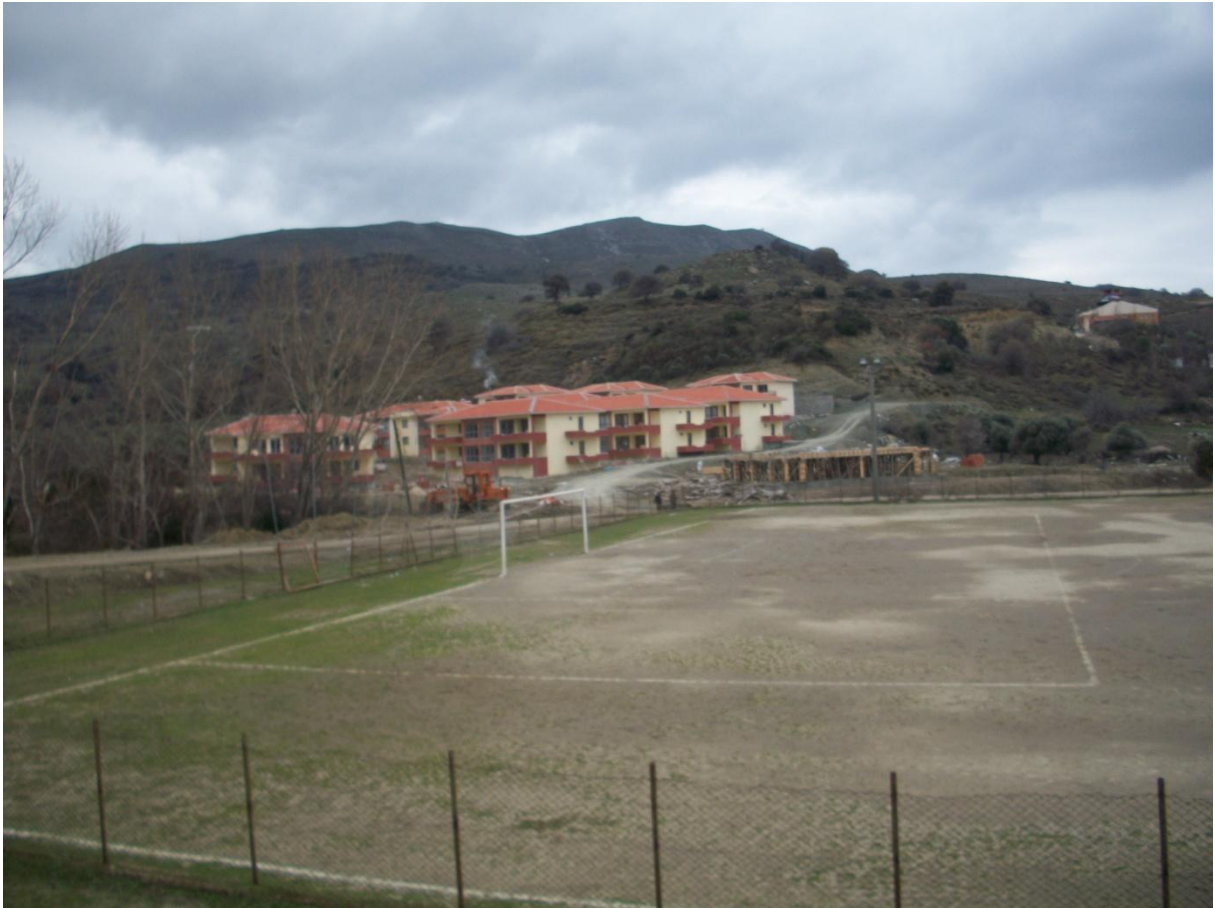
Photo 8. Unsustainable House Construction Near the Stream Bed (Gülbandılar, 2015)
