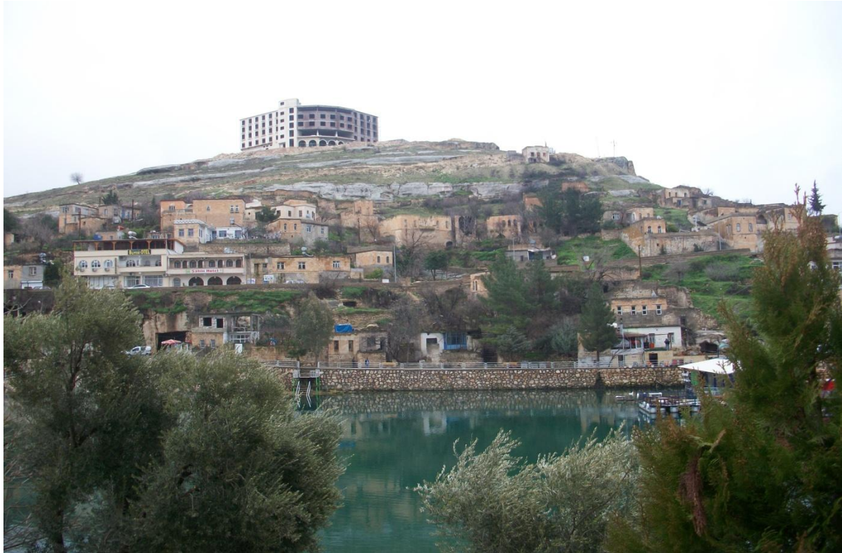
Photo 9. Ongoing Construction of Five-Stars Hotel in Halfeti (Gülbandılar, 2015)
