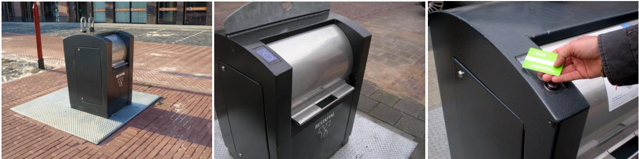
Figure 1: The underground collection system that residents use to dispose their residual waste. After scanning the key card it is possible to open the cover and put a bag of waste in the available space. When closing the cover the bag will fall into the underground container. Photographs by ROVA.
