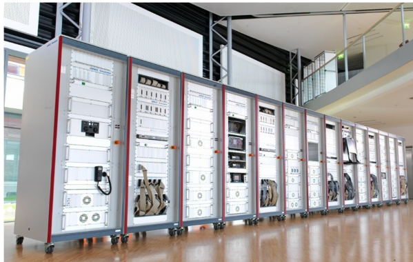
Figure 1.1: Ilab3 before installation
