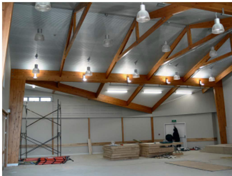
Figur 1.1 - Eastview Baptist Church Auckland (Manufactured by McIntosh Timber Laminates (now Timberlab Solutions Ltd))
