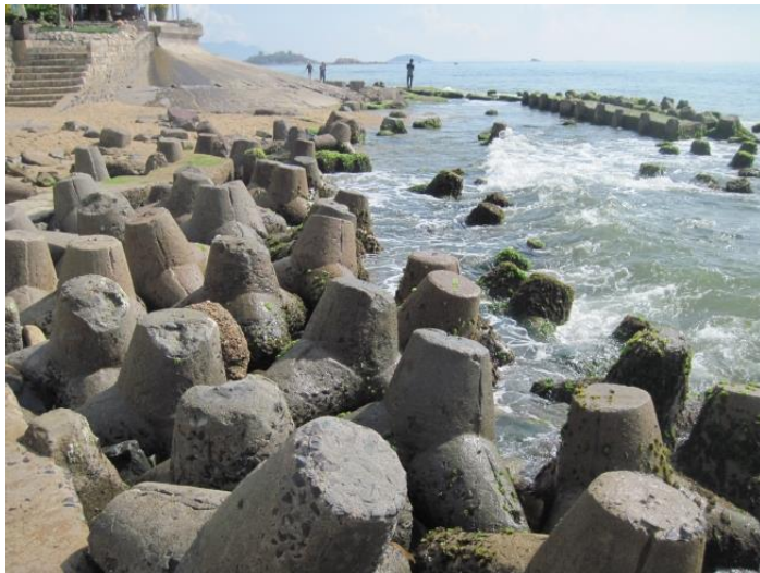
Figure 20. Two jetties made from tetrapods at the south of Nha Trang View restaurant.
