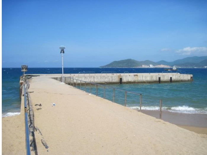
Figure 22. Vinpearl ferry terminal.
