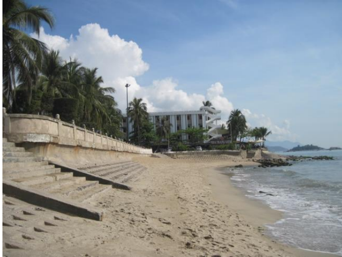
Figure 19. The seawall and the groins at the beach south of Nha Trang View restaurant.
