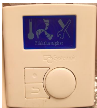
Figur 2 - Kontrollpanel ventilationsaggregatet.
