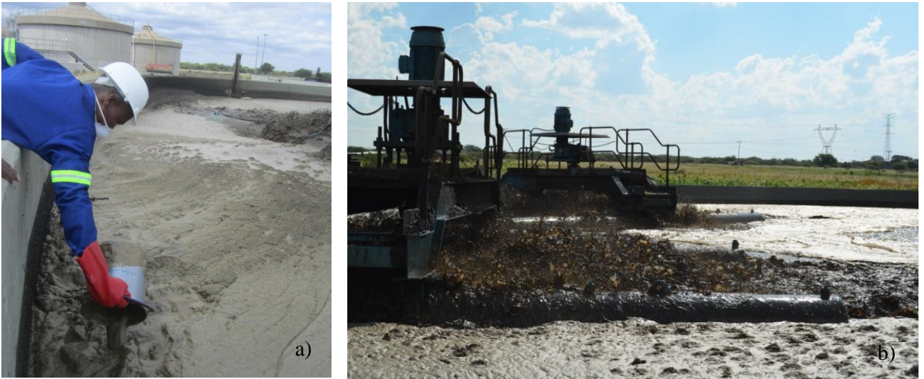
Figure 10.2. a) Sampling of secondary sludge from the aerobic digestion, b) Aerobic digestion tank
