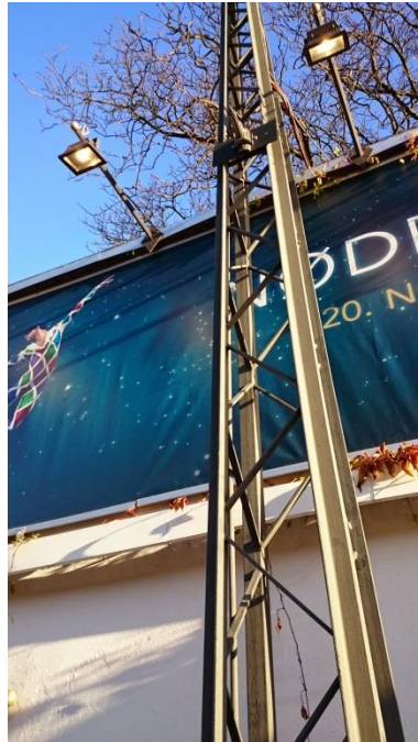
Figure 4-2 Framed structure found on many poles in Copenhagen
