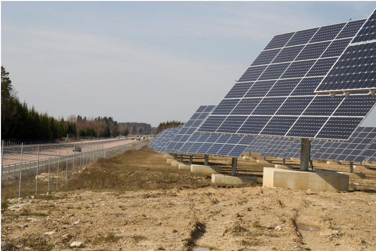
Figure 3-4. The solar park outside Västerås with modules on solar trackers. Picture taken by the author.
