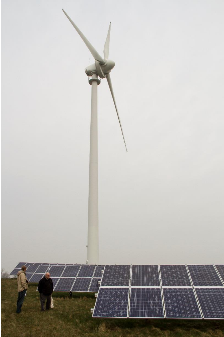
Figure 3-3. The solar park in Simris with a capacity of 442 kW. In the background, north of the park, a wind turbine also owned by Österlervind AB is seen. To the left is Henrik Davidsson together with the CEO of Österlervind, Ola Jönsson. Picture taken by the author.
