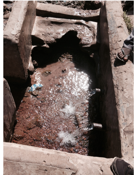
Figure 10. Spring well in Abolo Yero, Apac. The current state of some of the wells visited during the field study is in an acute need of reconstruction, as shown in the figure.
