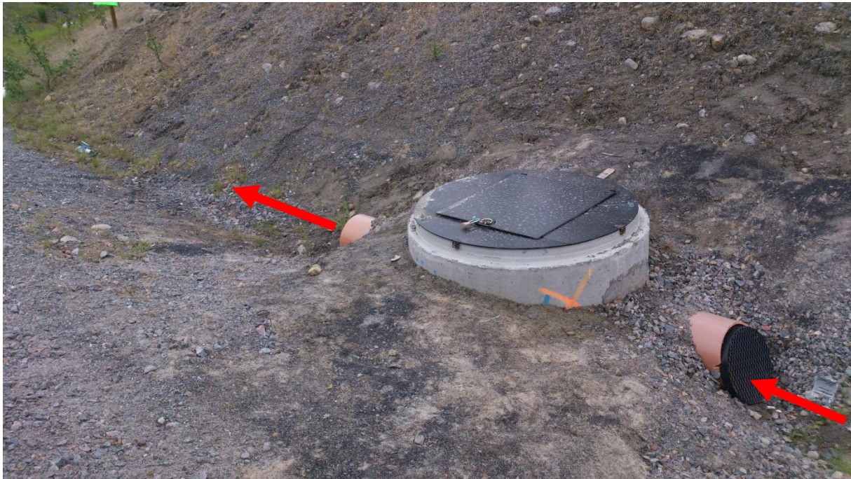
Figure 3. The flow measurement station in the downstream part of the swale. A continuous wave Doppler flow meter is installed inside the PVC pipe. The red arrows show the flow direction. Photograph by H. Rujner (personal photograph, June 11, 2014).
