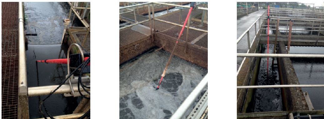
Figure 4.5. Pictures of online sensors for the measurement of suspended solids concentrations in (from left to right) the WAS, the mixed liquor of zone 5 and the SST effluent. 9 th of June 2015.
