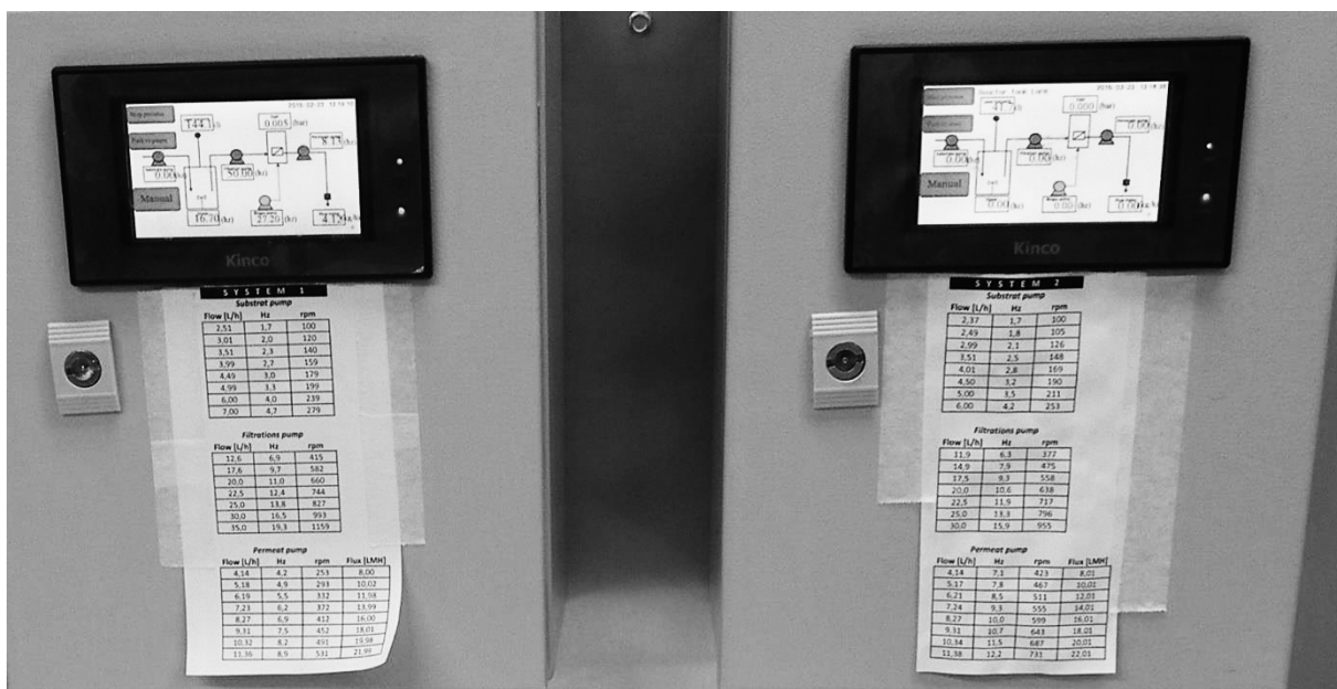
Figure 3-4. Control panels of both systems. Note that the left panel has red buttons and the right has green ones. These colors were alternated informing of filtration or relaxation mode.
