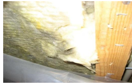
Figur 3.11 Mineralull, fuktskadad [61].
