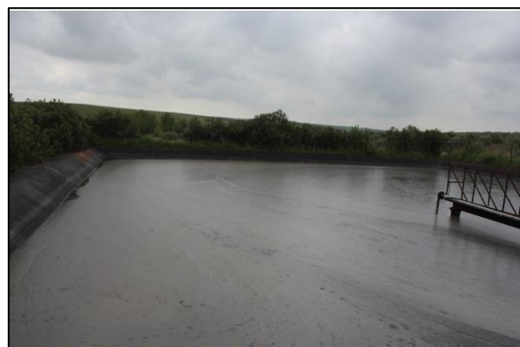
Picture 6: Aeration basins.
