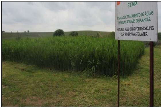
Picture 7: Natural reed beds to recycle wastewater.
