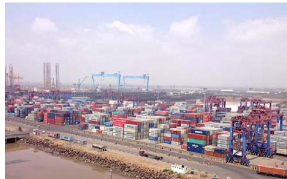
Picture 1 Port of Pipavav from Post-Panamax crane
