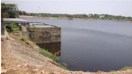
Picture 3 Water reservoir
