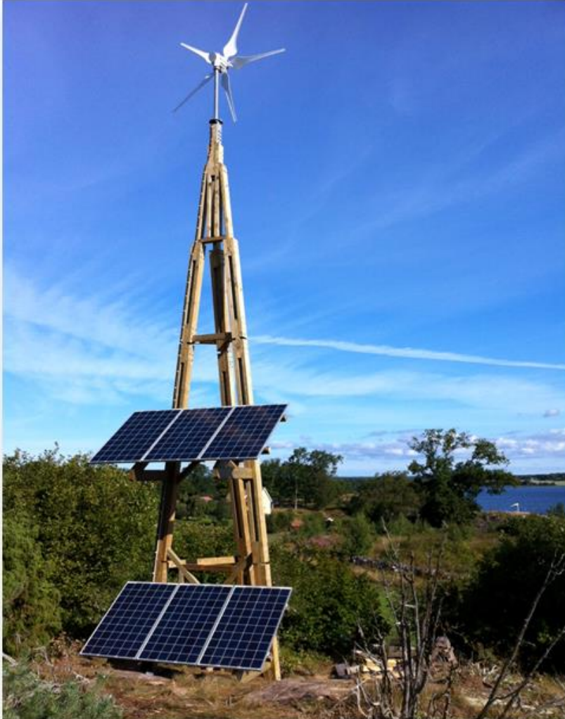
Figure 4. The Dali Powertower with 6 PV cells (Innoventum, 2014a)
