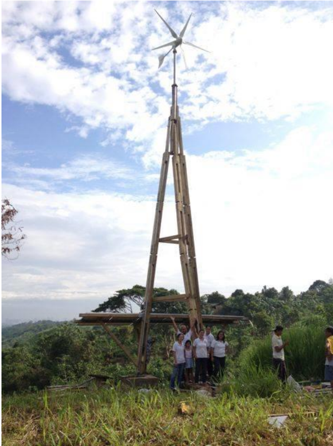
Figure 2. The PowerTower installed in Manila, the Philippines (InnoVentum, 2014b)
