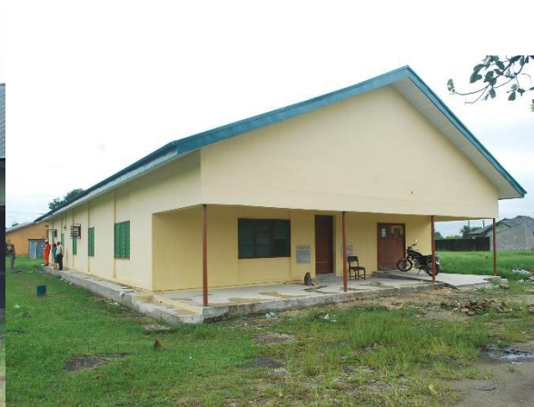
Renovation of Health Center at Ibenu
