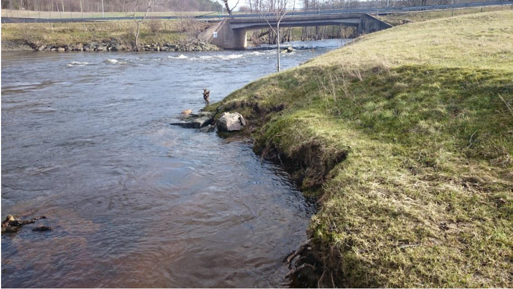
Figure 2.8: Săveân River within the study section showing erosion of the banks (Photo by Gasper Sechu)
