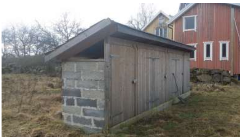
Figure 7: Chambered room to decompose human excreta (Photo by author, 2015).
