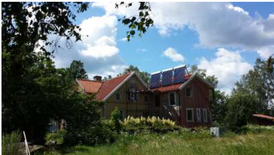
Figure 8: Solar Panels used for heating water mounted on the main house (Photo by author, 2014).
