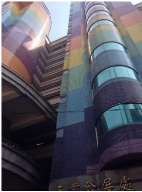
Figure 6. The old building
