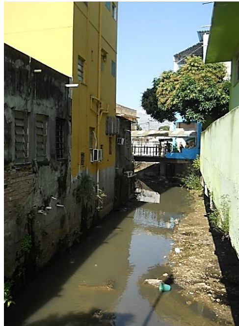
Figure 4.4 Illegal connections of sewage into Dona Eugenia River (Rezende, 2013).
